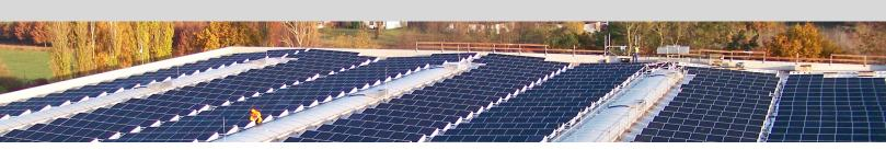
toughTrough GmbH developed a special penetration-free and low-ballast system for photovoltaic installations on flat roofs. Carefully performed analyses of conventional setup designs for photovoltaic modules revealed a great optimization potential, especially regarding mounting systems. Additional wind tunnel tests, simulating environmental conditions, provided detailed data about the aerodynamic characteristics, such as the impact of wind loads on the modules.
